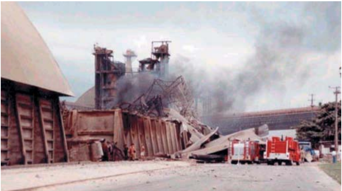
Figure 3: Warehouse of the company Coimbra after the dust explosion (credit: Cris Coutinho)
