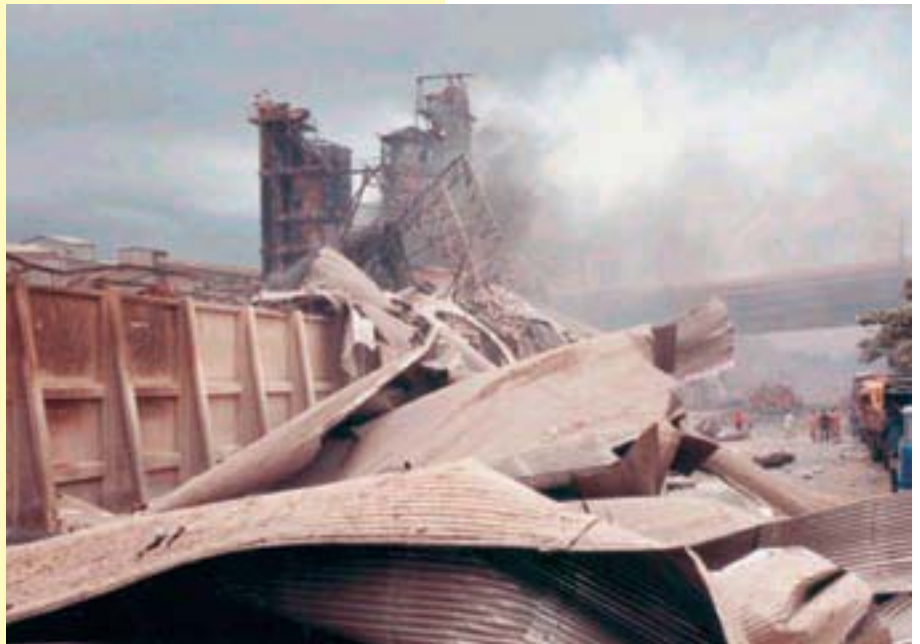
Figure 1: Result of a dust explosion with extreme destruction (credit: Cris Coutinho)
